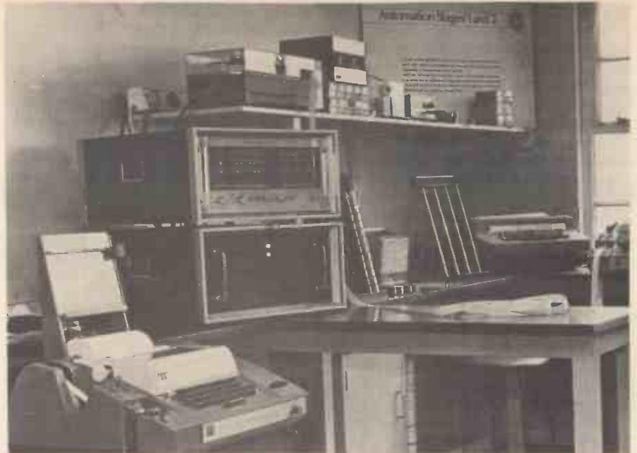
*A Minic Computer in use at the laboratory of the Government Chemist. For analysis of the weight and moisture content of cigarettes and tobacco. This all-British computer was one of the first to use the "firmware" concept, in which the programming is simplified*
