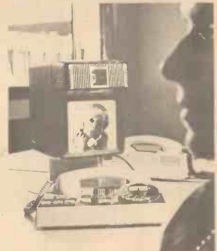
The new videotelephone retains the three original functional units: the telephone, the picture unit and an attachment box. There is a button for hands-free conversation and a volume control switch. The picture unit is rotatable, and its camera section can be tilted. A mechanical scissor aperture permits the use of plumbicon and silicon-vidicon type camera tubes, as well as the conventional vidicon.
