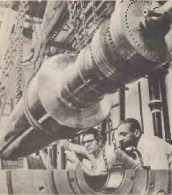
Fig. 16 Prototype 5MW superconducting rotor of a power generator made by Westinghouse.
