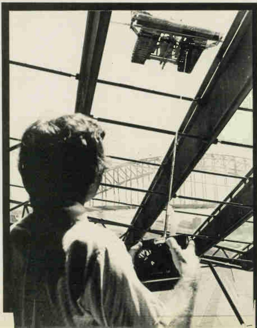
were startlingly effective. Traction was excellent. Successful cleaning demonstrations resulted in an order for three tractors, (one for each roof and one spare) thus successfully completing a remarkably farsighted and difficult project.
