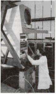
Vibration testing: a sophisticated vibration and shock testing system can take anything from elecronic components to assemblies of up to 2 tonnes in weight. (Seimens Plessey Assessment Services Ltd., Fareham.)
