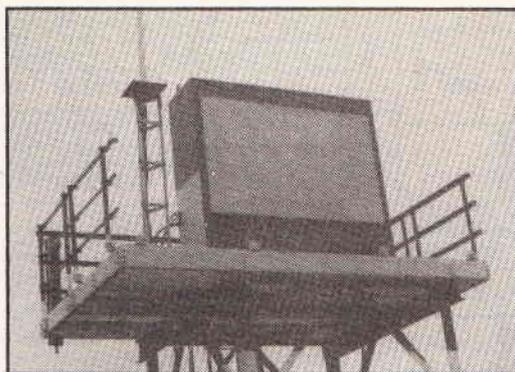
Fig. 11 The Azimuth transmitter of the MLS installation at Port Hawkesbury, Nova Scotia. The equipment is mounted on a tower to ensure coverage over a hump in the runway. The vertical aerial to the left of the main array is for Distance Measuring Equipment which gives the aircraft its distance from touchdown.
