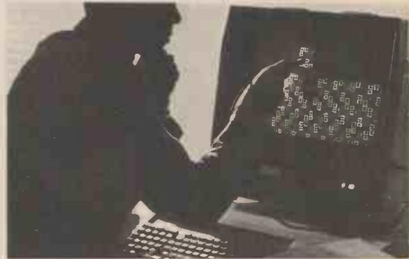
**Designer in dialogue with computer.** A senior designer is shown adding another stage to the MOS microcircuit which he is designing in co-operation with a Myriad computer. He is using a light pen to put a new section into the main circuit design, having called it from the computer store using the keyboard. (*Marconi*)
