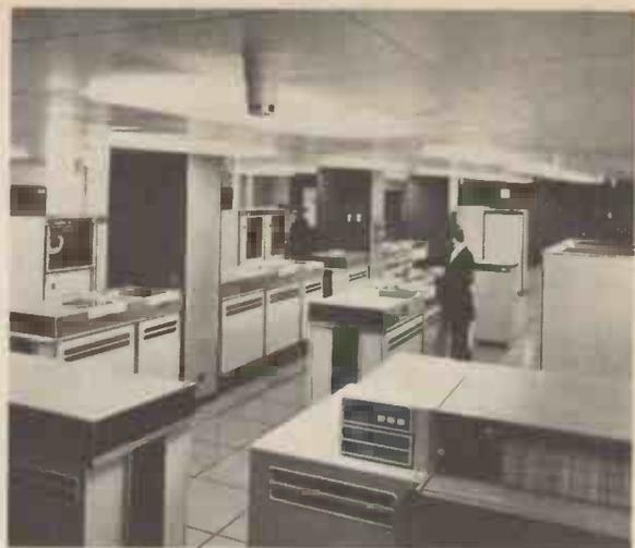
A finance company uses this large computer installation for the maintenance of the accounts for customers and dealers. The system uses a variety of peripheral devices, including a high speed printer, magnetic tape drives, magnetic disc drives and a paper tape reader. (*The National Cash Register Company Ltd.*)
