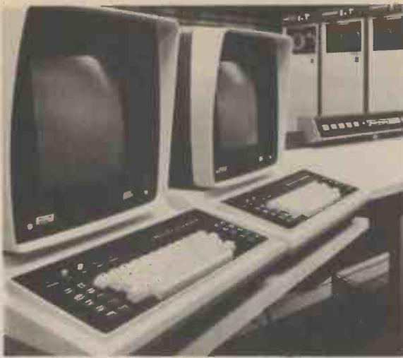
A pair of visual display units are shown here against a background of magnetic tape drives. Information is shown on the face of a cathode ray tube, as in a television set. (Burroughs Machines Ltd.)
