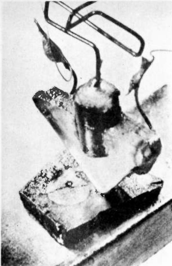
Photograph of the first original semiconductor amplifying device—the transistor.
