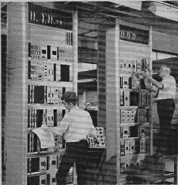
The first pulse code modulation tandem exchange relays record the digits you are dialling. (Post Office)
