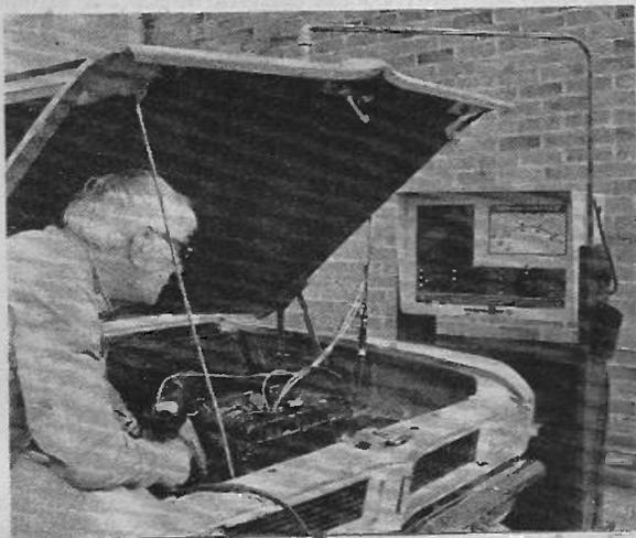
The Crypton "Motorscope" Mk VI—engine analyser shown in use.
