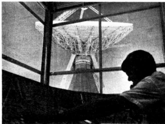
Part of the control console and, through the window, the antenna of the satellite earth terminal in Bahrain. Part of a world telecommunications network, it was built by Marconi and is operated by Cable & Wireless.
