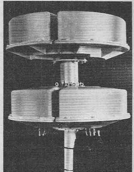
Double cake shaped aerial of Decca's EW equipment. Being designed to fit around a mast, it does not compete for the sought after masthead position.
