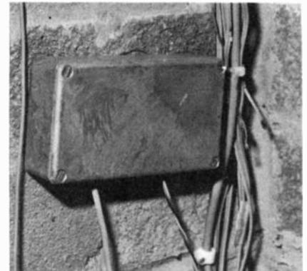
Ultrasonic Receiver (item 4) mounted on inside wall.
