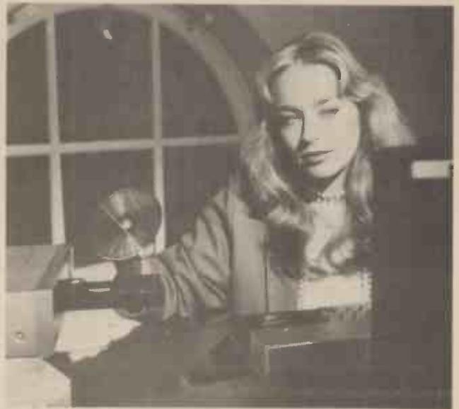
*Philips latest information-storage medium consists of a Philips MSX computer, CD player, video monitor and Software. Future CD systems will allow all kinds of text, graphic and sound information to be stored and combined. The function of the computer is to enable information to be accessed selectively.*
