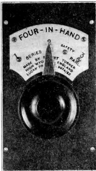
It is often very useful to be able to switch over one's aerial condenser from series to parallel, but the advantage is trebled if by so doing an overlap in wave-length can be obtained without altering the aerial coil. This fact has been realised by Mr. Ernest Turner, of High Wycombe, who has patented an arrangement a back and front view of which is reproduced herewith.
