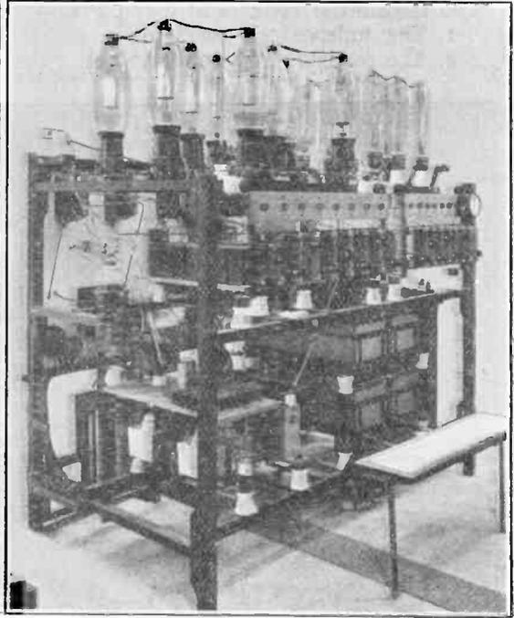
Fig. 7. Rectifiers and power valves.
