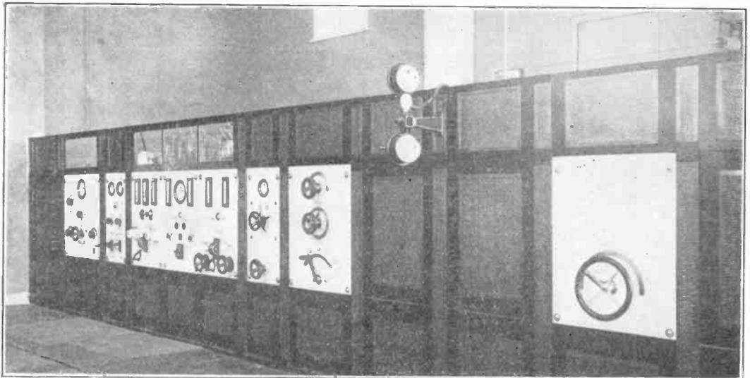
Fig. 5. Panels of the 14kW transmitter.
