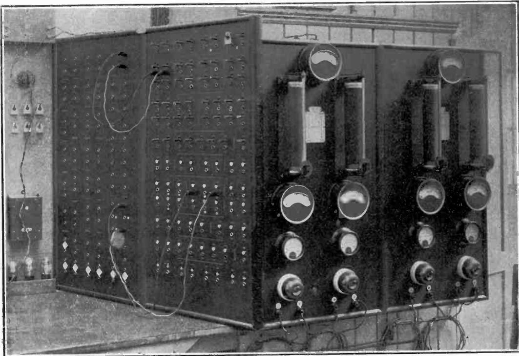
Showing the battery supply panels and charging board.
