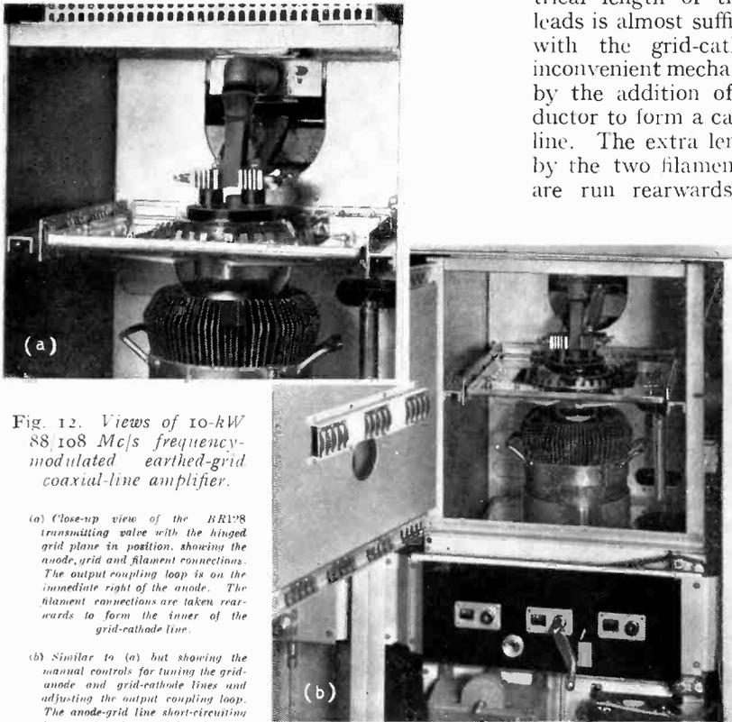
Fig. 12. Views of 10-kW 88-108 Mc/s frequency-modulated earthed-grid coaxial-line amplifier.
