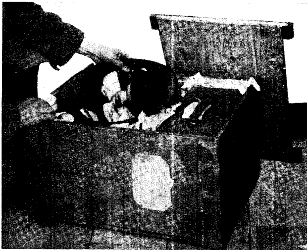
Fig. 3. Loud speakers need very careful packing. The illustration shows how the instrument and trumpet are included in the same case. Paper is used as packing material
