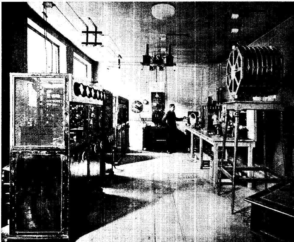
CONTROL ROOM AT THE RADIOLA STATION
