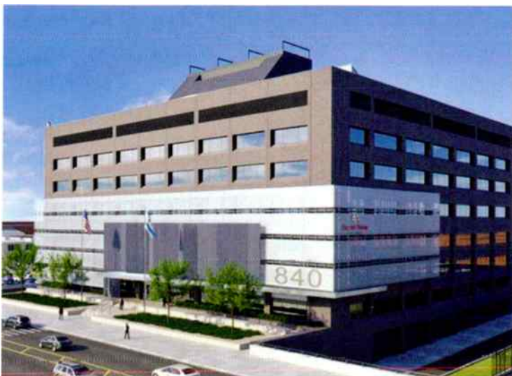
Server Farm Realty's new 450,000 square foot data center in Chicago. Cloud servers feeding the internet are where music is stored nowadays.
