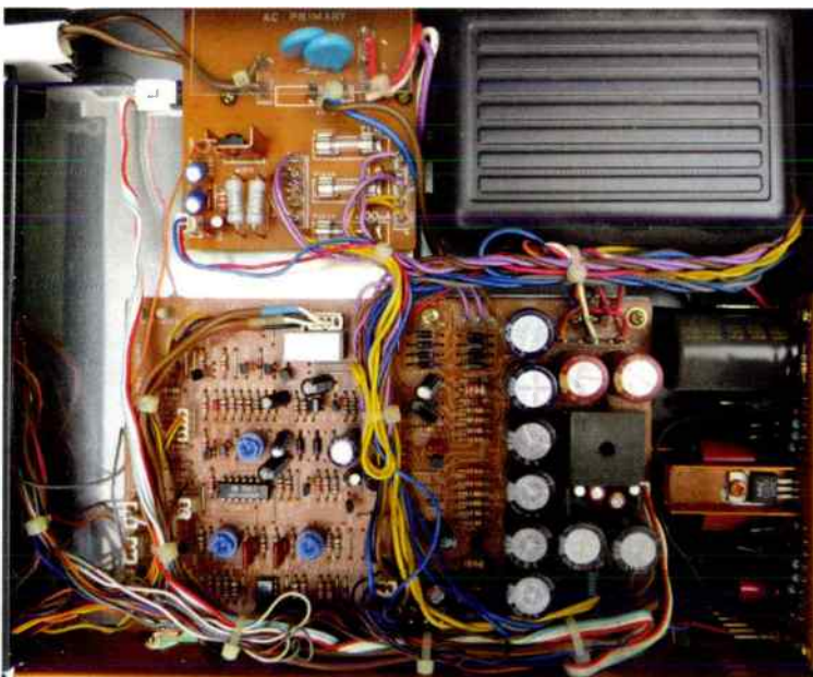
All that complex circuitry needed a beefy 40 Watt power supply, built around the large screened transformer visible on the top-right. The silver box occupying the left contains the digital circuitry that converts the digitised audio into video. This too was screened to prevent noise from contaminating the analogue audio.
