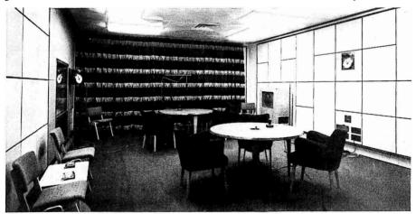
Fig 11. Modular acoustic treatment in Broadcasting House Extension.
