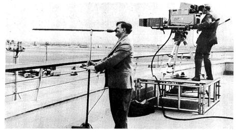
Fig 8. The "rifle" microphone being aimed at an aircraft to provide close-up sound for a TV broadcast.
