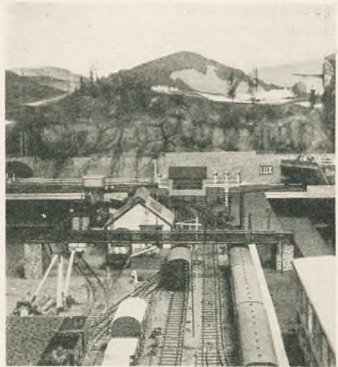
Extension lines at station on the North Midland Railway. The metal yard crane and loading gauge can be seen.
