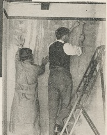
Fixing up the boards
