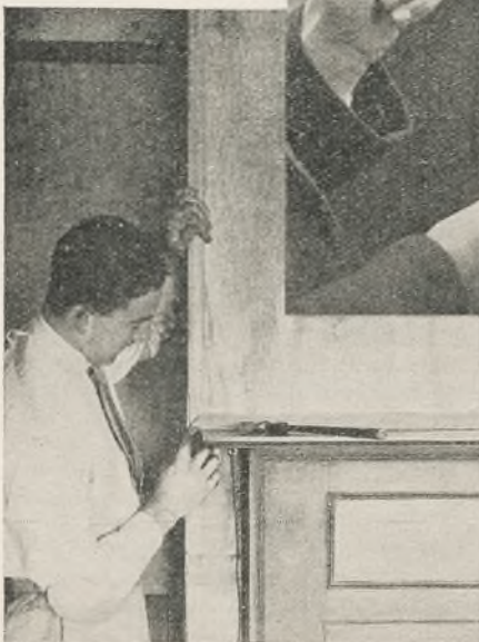
Fitting a mitred corner
