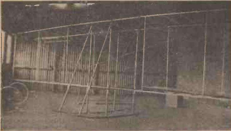
This photograph shows the uncoversed framework of the completed glider.
