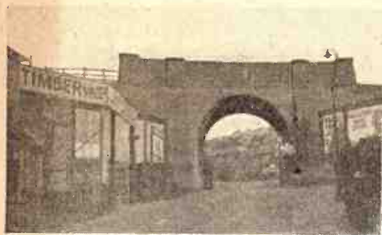
A simple Semi-circular arched bridge over road
