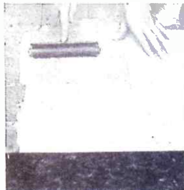
Using a squeegee to set the tile and remove any underlying air bubbles
