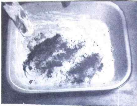
Mixing the cement with colours. Note they are laid across the plain mixture in separate lines
