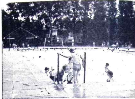
A happy place like this may quickly be transformed into a scene of tragedy where a life could depend upon a prompt rescue.
