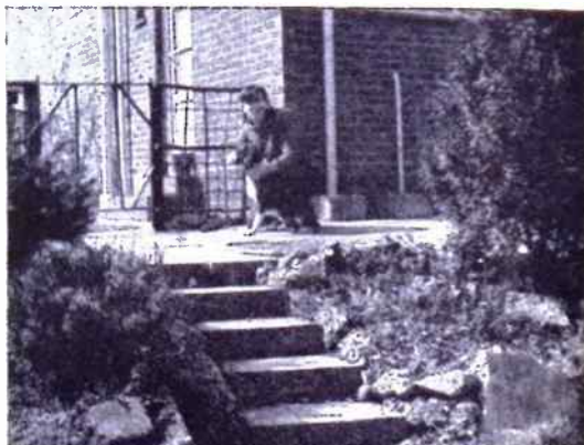
Fig. 2—Cement steps, the inner core of which is composed of broken bricks and stones mixed in with the cement
