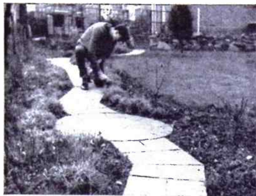
Fig. 1—Cement path marked out with straight edge. Variety is given by a circular slab and different angles
