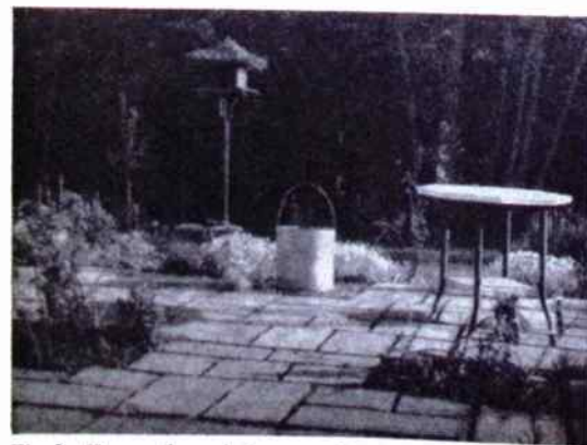
Fig. 3—Terrace formed of separate blocks made by using strips of wood, removed when cement has set
