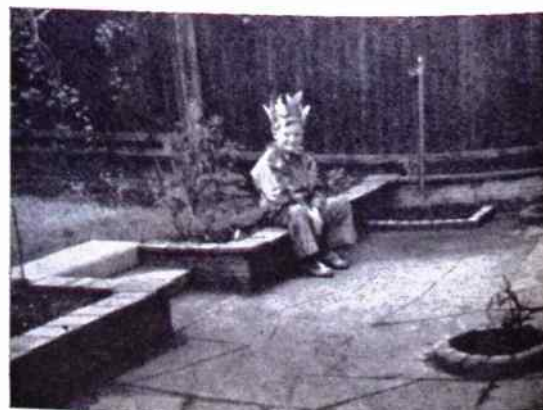
Fig. 4—Showing low retaining walls marked out in various ways. Curved walls are made with the help of strips of linoleum.
