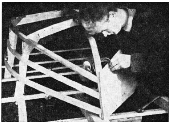
Fixing the first side panel. The lengthwise parts are fixed to the stem and rest in the former slots
