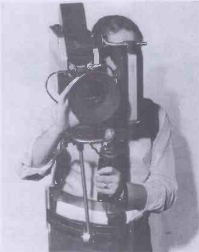
*A Philips 'Minicam' attached to a cameraman. The collection of straps and links ensures the maximum manoeuvrability with the minimum of strain on the operator.*
