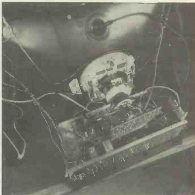
Rear view of Ferguson colourstar TV, 1968. This was the first all-transistor colour TV in the world, and it uses a 25" (635 mm) Thom-Mazda tube. It features modular construction: printed-wiring panels are removable for easier servicing. It was manufactured by Thom Consumer Electronics in Enfield, Middlesex
