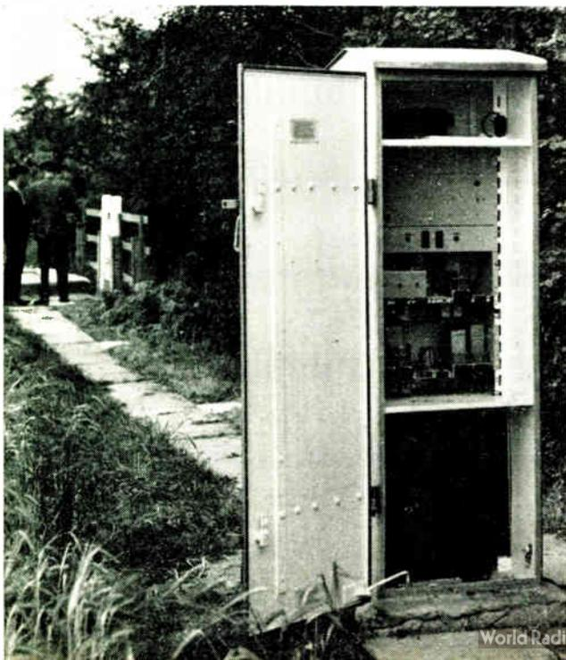
been installed in England on behalf of Shellmex and B.P. Pipelines Department to operate motorized valves at isolated points along an oil pipeline. Hitherto, staff have had to travel long distances daily to adjust the valves by hand; adjustments can now be made for the cost of a telephone call and emergency action can be taken within seconds.
