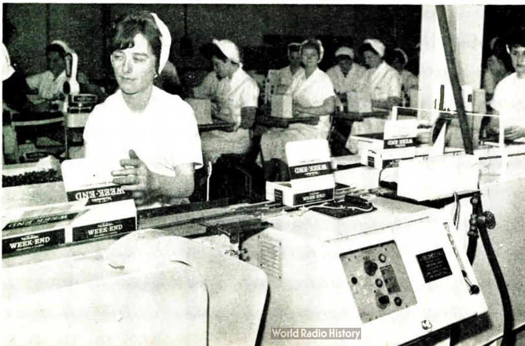
◀ *Another MC200 in action. At John Mackintosh's confectionery factory at Norwich underweight boxes are pushed to the far side of the belt by a ram. This section is cordoned off and the underweight cartons are made up, reweighed and returned to the production line*
