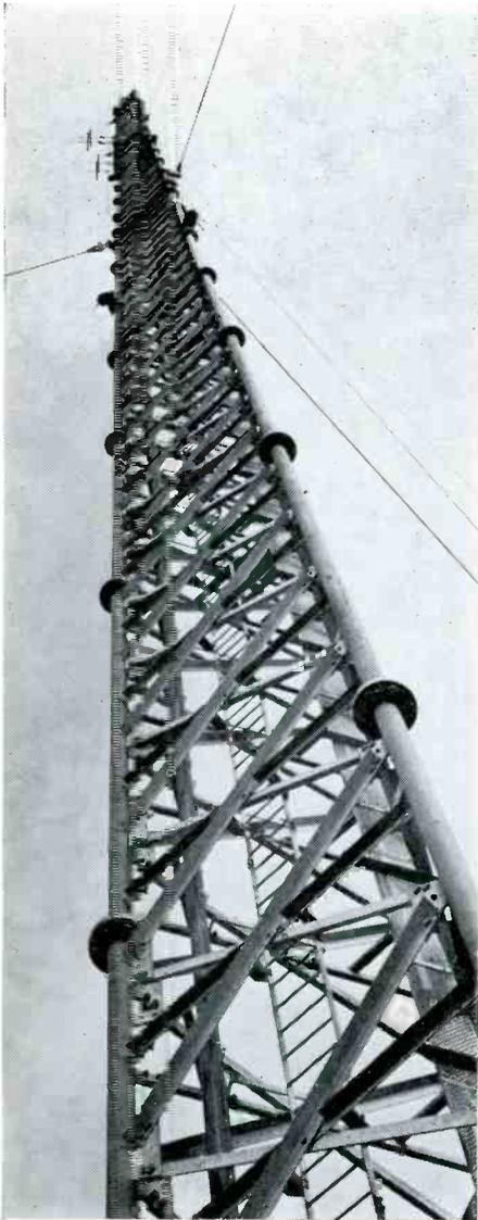
The new 750 ft lattice television mast at Rumster Forest, Caithness, designed, supplied and erected by British Insulated Callender's Construction Co Ltd to the order of EMI Electronics Ltd for the Independent Television Authority. It was erected by a team of eight men and is the most northerly ITA mast in the United Kingdom. The Station came into service on June 25 and transmitted Grampian TV programmes on Channel 8 over an area which includes the Orkneys.
