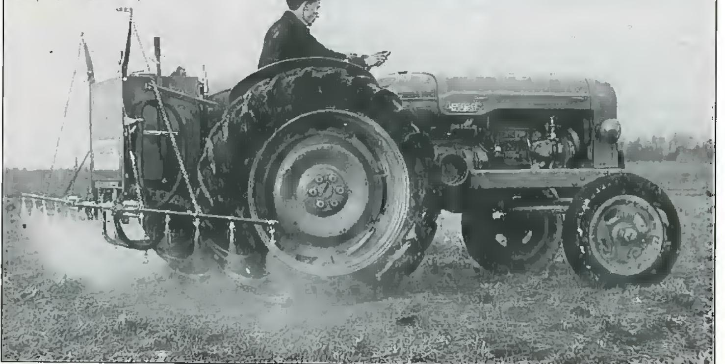
weed coverage was no longer necessary, the volume of spray could be reduced from 100 to about 20 gallons/acre. Moreover, as the newer herbicides were applied as a solution, the need for mechanical agitators in the sprayer tank was eliminated. Sprayer design was enormously simplified and this spawned a new generation of 'low volume' farmer-owned spraying machines; it was a classic example of a new chemical bringing about a revolution of crop spraying technology.
