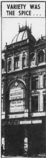
The Bedford Theatre—Your Own Family Showhouse—the sign still stands out in Cromwell Road. But the music hall has been derelict since it was closed in 1950.
