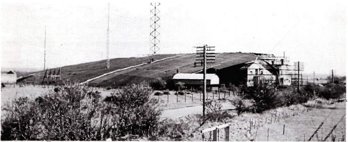
The station with partially completed camouflage.
