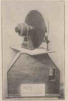
This photograph shows the synchronising motor, disc and television lamp.
