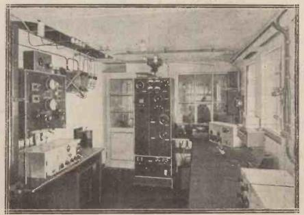
The short-wave transmitter (centre) on board the German liner "Bremen." The receiver is shown on the left.
