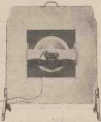
The back of the Fire-Screen Cone, showing the essential simplicity of the arrangement.
