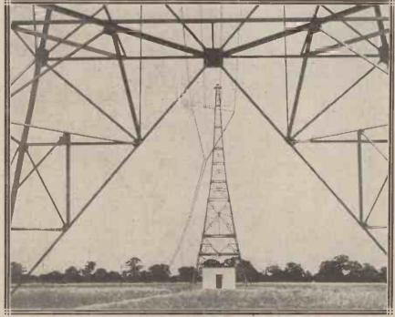
One aerial system of the new 2 LO, seen from under one of the masts. The building shown houses the complete aerial tuning equipment, which is supplied with H.F. by means of a feeder line connecting it with the main transmitter in the main building.
