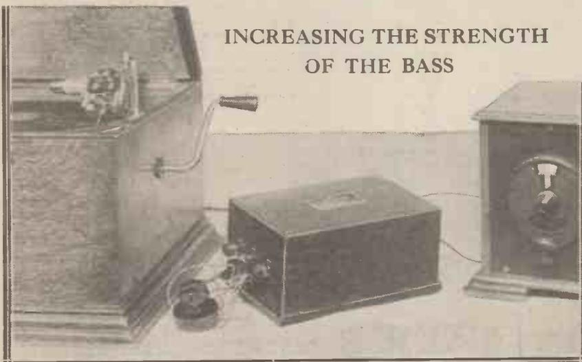
The Gam-brell "Novotone" in operation with an ordinary set. Note the 30-ohm variable resistance for reducing scratch.
