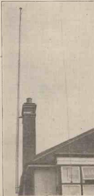
A down lead terminating in a lead-in which goes directly through the window frame.
