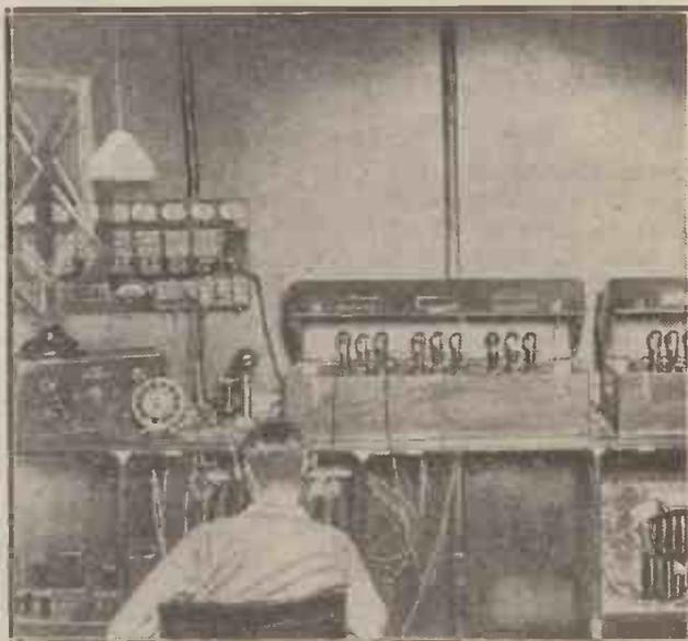
Part of the home-made radio outfit used at Sing-Sing Prison to supply broadcast programmes to the 2,300 'phones and 21 loud speakers installed in the buildings and cells.
