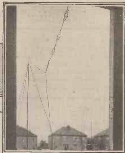
A PROPERLY arranged outside aerial is a lightning protector; providing a lightning arrester and/or an earthing switch is fitted, the aerial conducts all dangerous atmospheric charges direct to earth. This fact should be universally known by now, but there are still a few
