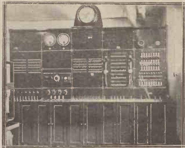
Above we have control board No. 2, which contains measuring and control apparatus for the amplifiers, the switching for outside broadcasts and lines to the relay stations. (Left) a general view of the huge new Broadcasting House.
