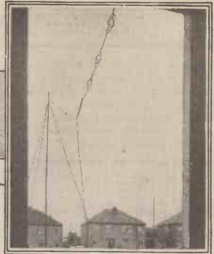
A PROPERLY arranged outside aerial is a lightning protector; providing a lightning arrester and/or an earthing switch is fitted, the aerial conducts all dangerous atmospheric charges direct to earth. This fact should be universally known by now, but there are still a few
