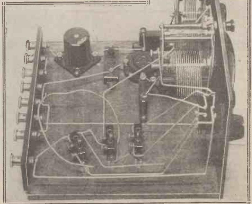
The two flexible leads in the foreground of this photograph are for the tapplings on the two "X" coils. The centre coil holder is the supplementary reaction coil.
