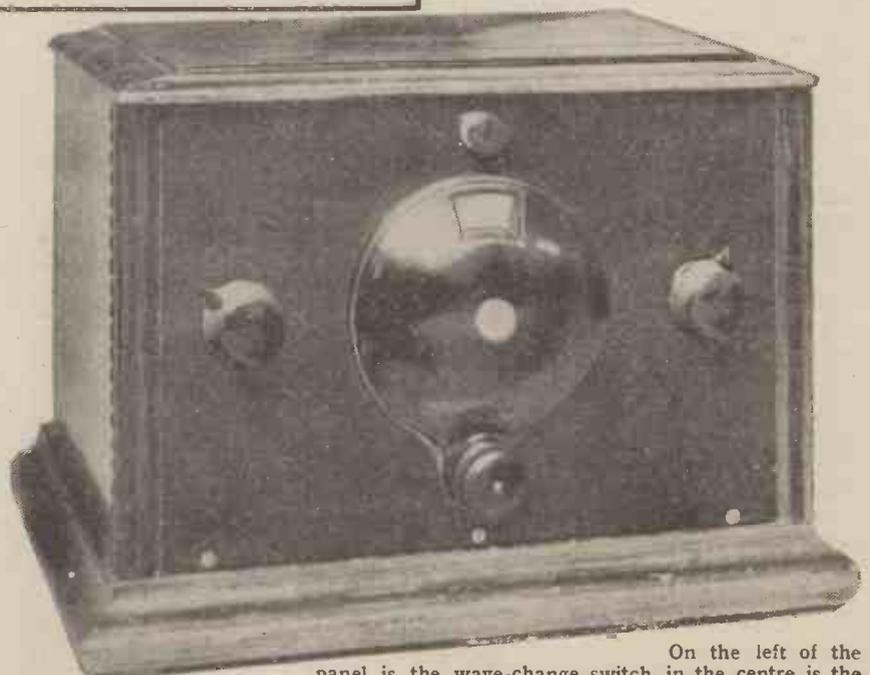
On the left of the panel is the wave-change switch, in the centre is the tuning control, and on the right the reaction condenser. The remaining knob is that of the on-off switch.
