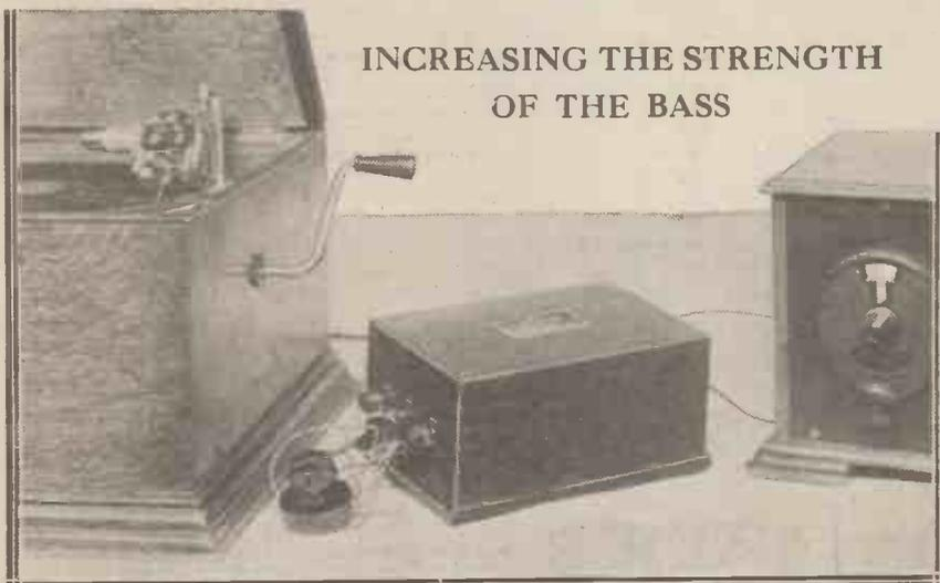
The Gam-brell "Novotone" in operation with an ordinary set. Note the 30-ohm variable resistance for reducing scratch.
