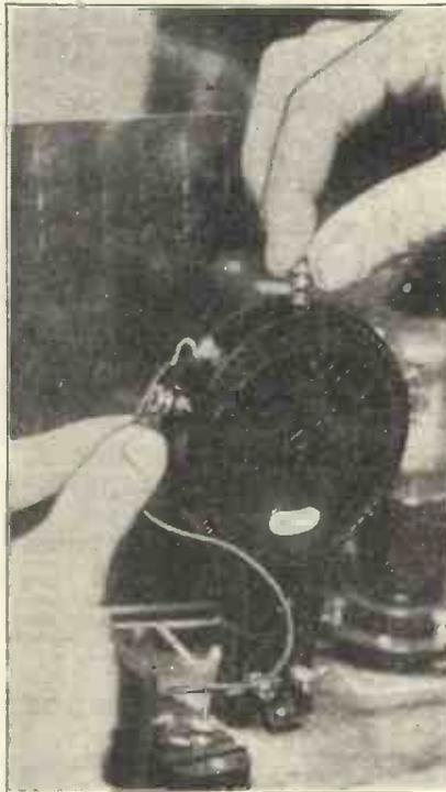
This point is important! In joining up baseboard "X" coil holders the pin should be connected to that part of the wiring that goes to earth. This is because the tappings on the coil are nearer the end of the winding which is joined to the socket on the coil mount.
