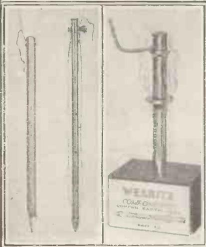
Three earth pins—excellent "anchoring" for your set. The one on the right has a novel soldering system.
