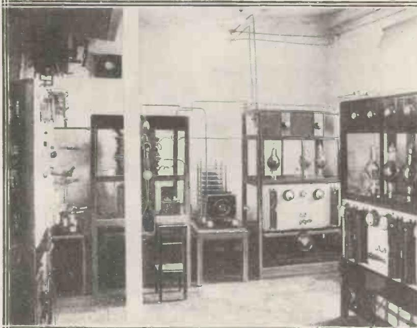
This is the transmitting apparatus at the Seville station. It has a power of about 1½ kilowatts, and shares the wave-length of 368.1 metres with the powerful Helsinki station. For this reason it is audible in the British Isles only when the latter transmitter is closed down.
