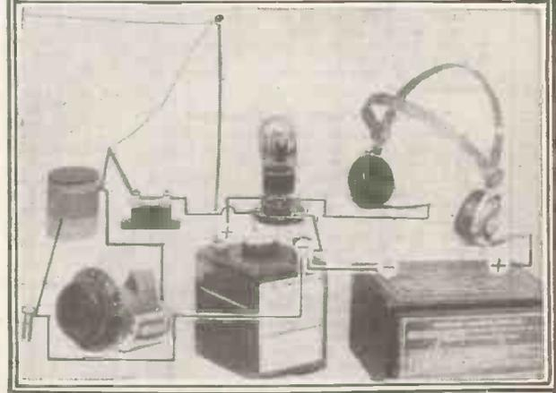
The voltages on the grid vary the anode current, and the grid leak and condenser cause detection (rectification).
