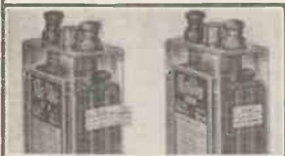
A couple of Exide two-volt accumulators of average capacity.
