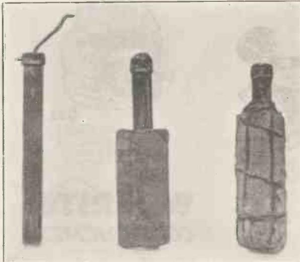
First we have (left) the central carbon rod, and then you see the carbon rod fixed in the bag containing the depolariser, around which a sal-ammoniac paste is packed. Two different types of bags are shown.
