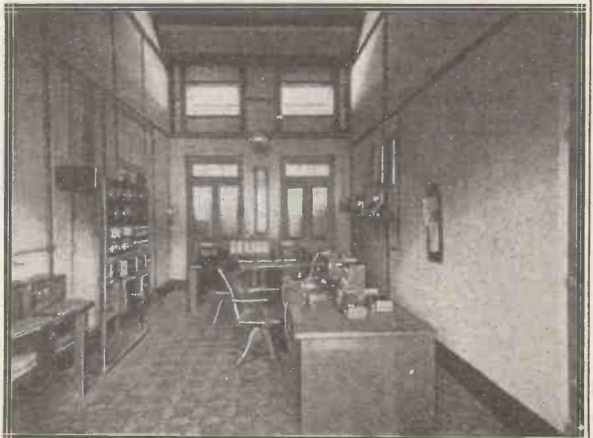
This is the main control desk (foreground), with standard receiving sets on the bench to the left, near the switchboard.
