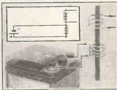
Current passing through the first coil sets up a field of magnetic influence which envelopes the second coil. Current is induced in this second coil every time the magnetic field changes in intensity. In the above case the switching on and off of the battery produces the effect.
