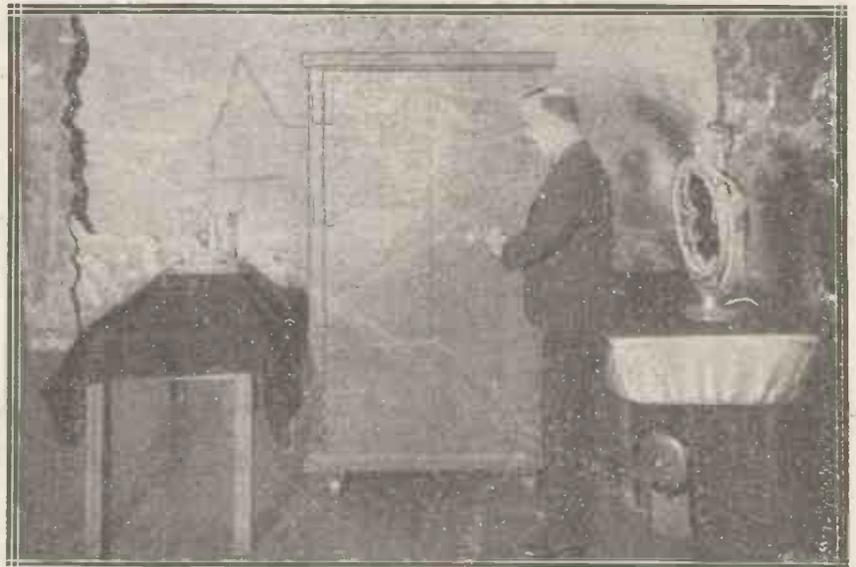
Invisible rays of light pass across the front of the safe seen above, and the little instrument to the left works burglar alarms if anyone cuts off the rays by going near the safe. This scheme was employed at a recent London exhibition to protect a particularly valuable exhibit.
