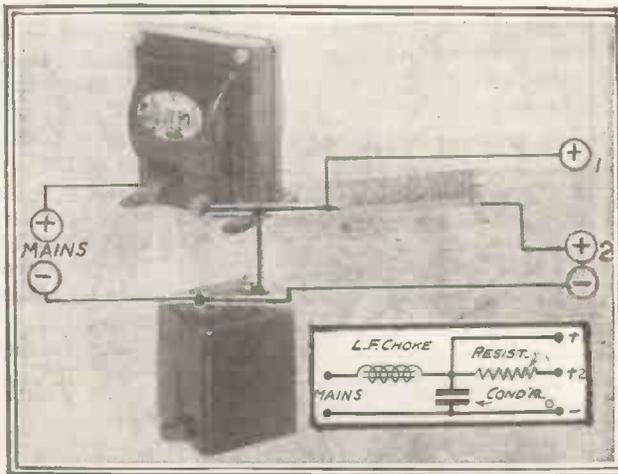
Smoothing mains current so that it can be used as H.T. for a set by taking advantage of the varying degrees of opposition offered by a condenser and an L.F. choke.
