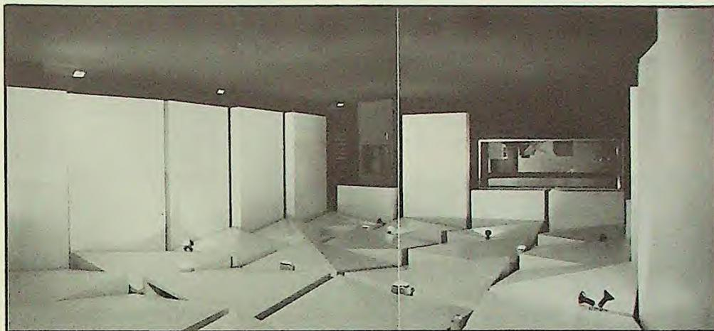
THE STUDIO interior with control room (left) and door to separation room (right). The wall and ceiling soundboxes were specially designed by Ken Shearer for Eden.
