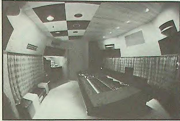
*“SUPER BEAR . . . Pride of place in the control room is an MCI JH-500 automated console equipped with 28 input channels, 32 outputs and plasma display monitoring. Tape machines are also by MCI: track laying is handled by a JH-16 Series 24-track with varispeed, and two 2-track and one 4-track are on call for mastering.”*
