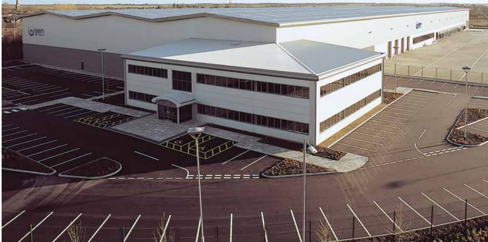
ABOVE Doing the Raunds | Gem has invested £15 million into its giant warehouse
