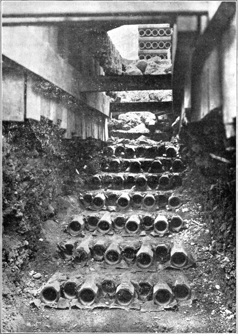
FIG. 2.—ST. PAUL'S CHURCHYARD. FORMATION OF NEW DUCT LINE.
