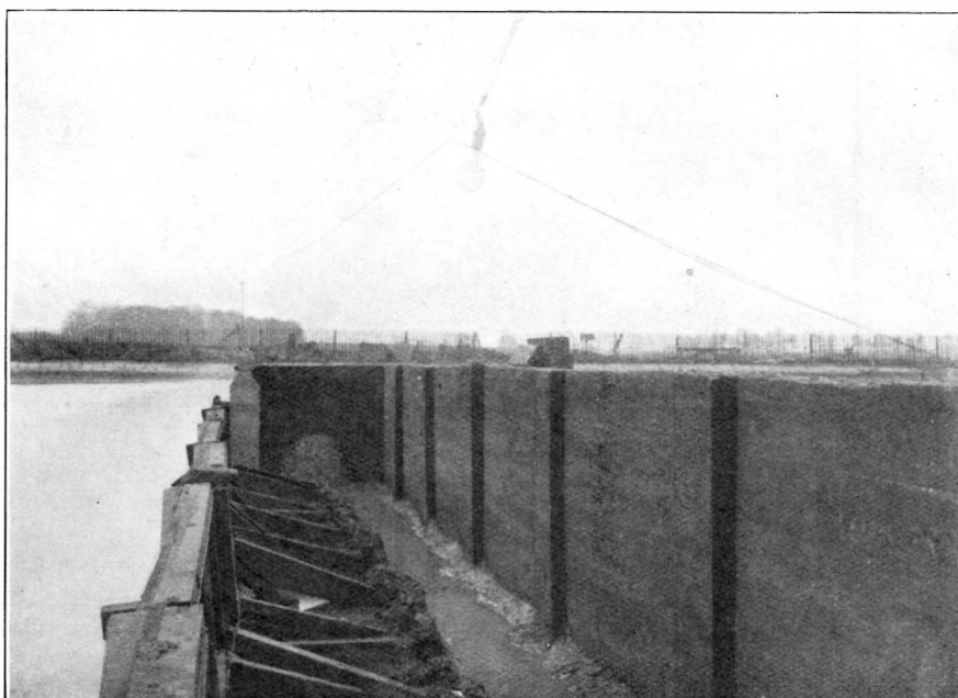
FIG. 4.— THE DAM AND ITS STRUTS.
