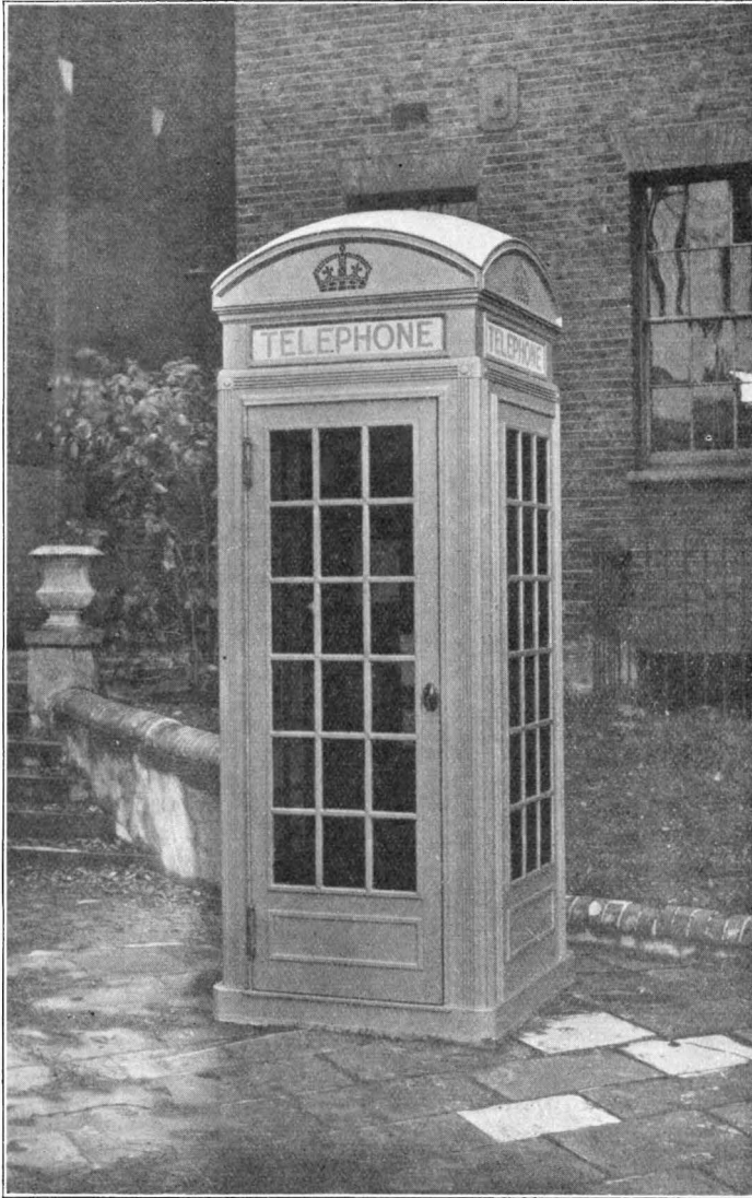
FIG. 1.—CAST IRON KIOSK: DESIGNED BY SIR GILES GILBERT SCOTT, R.A.
