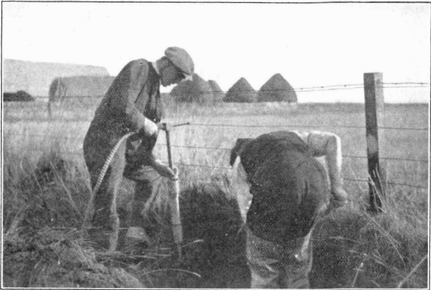
FIG. 6.—TRENCH DIGGER 158 IN OPERATION.
