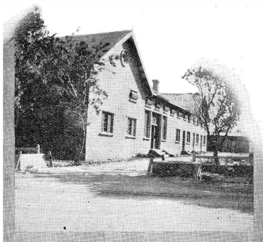
QUETTA PUBLIC EXCHANGE BUILDING
