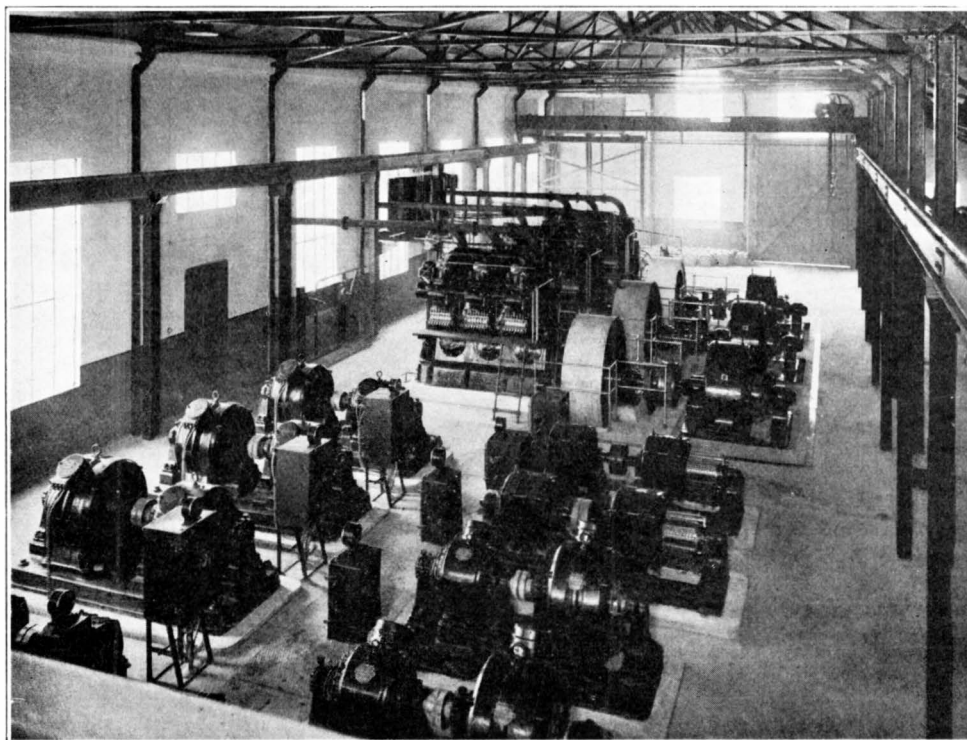
FIG. 2.—BODMIN ENGINE AND MACHINE ROOM.
