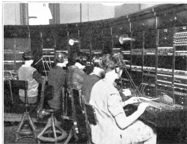
FIG. 7.—MANUAL SWITCHBOARD, HANLEY.
